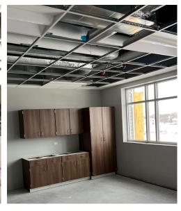
The coming months will see a series of finishing touches throughout the building. Classrooms will soon be illuminated with newly installed light fixtures, adorned with Acoustical Ceiling Tile (ACT) ceilings, and outfitted with completed casework, interior glazing, and doors.
